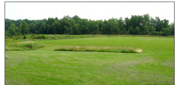
PHOTOS: EXISTING DRAINAGE FOR SURFACE RUN-OFF FROM THE SCHOOL BUILDING AND PARKING LOT
